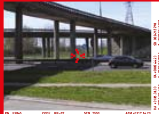
Infrastructure & Road construction
